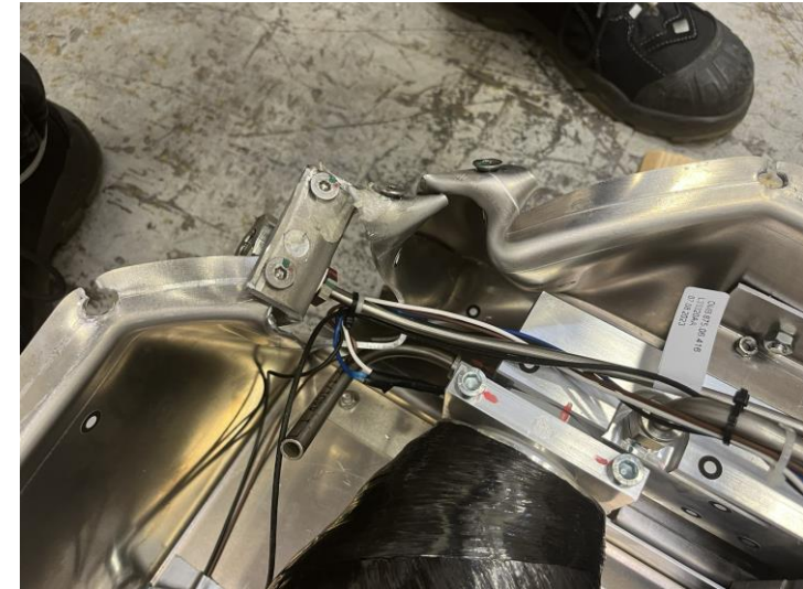
Significant plastic deformation of piping
