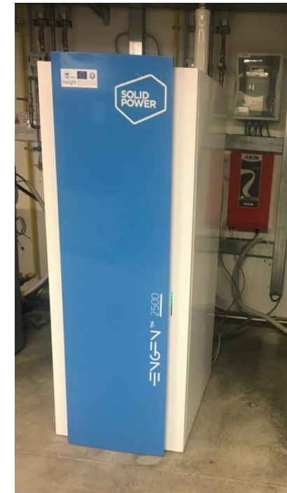
Figure 17- Final system installed on field.
